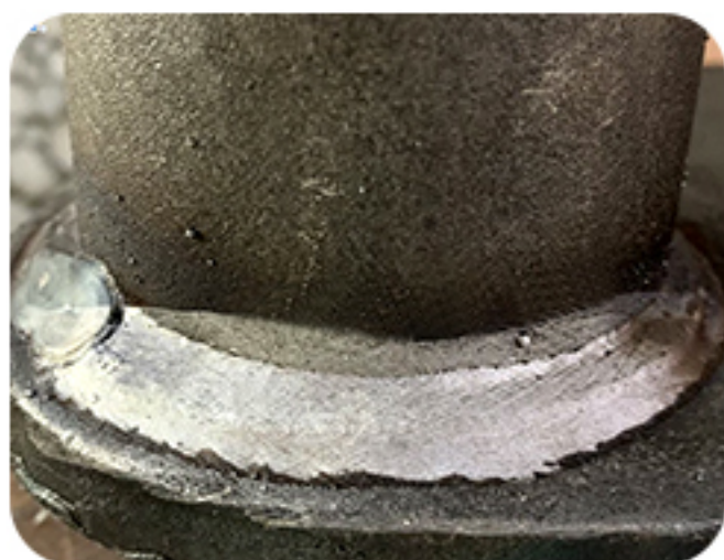
Weld Seam Cleaning
